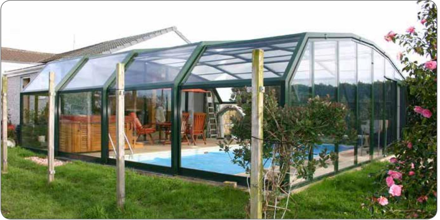
This model of the telescopic swimming pool enclosure retracts back towards one end and is mainly sold in warmer climates with constant sun such as the south of France, Spain or Italy, where one opens his enclosure only once a year. It can also be used in other areas, if the enclosure is attached to the house with all sections retracting back towards the rear. Planning permission is normally required in that instance.
