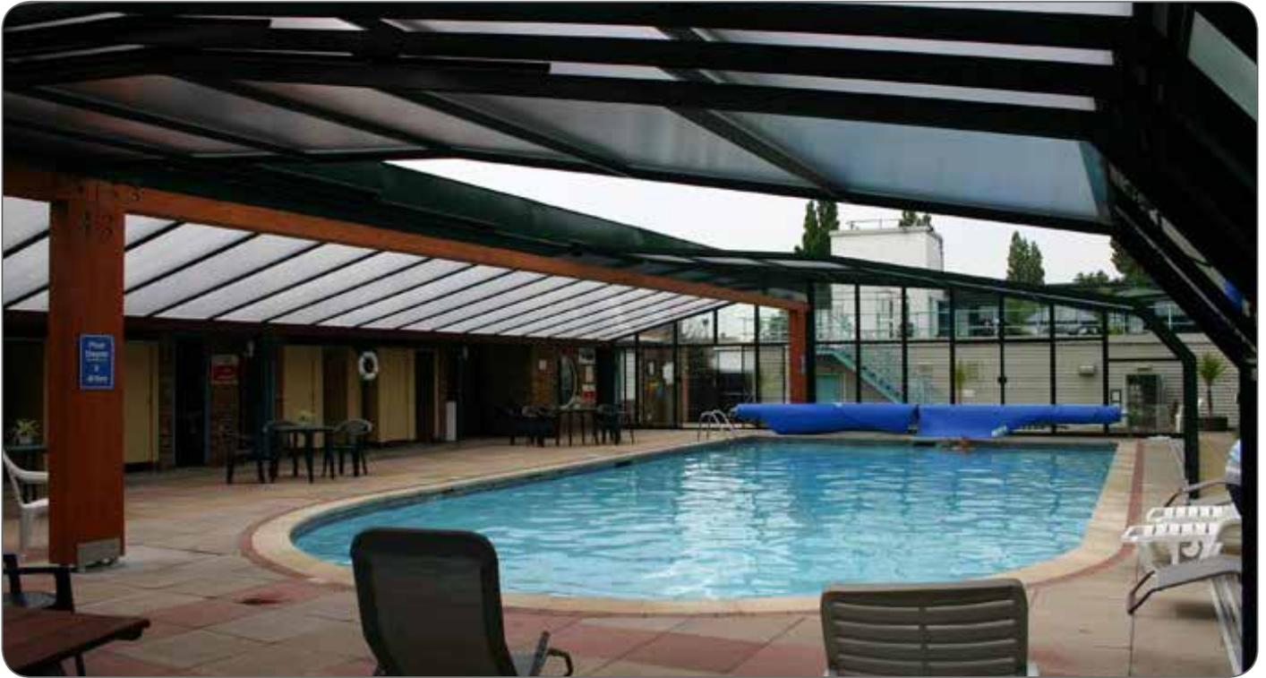
We manufacture the superior quality that consists of aluminium profiles in high-quality alloy with a basis of manganese and silicon (ref. 606035 T6 F22S) of an increased resistance and of a weight of  $\pm 2,3$  kg/m for the carrier profile.
